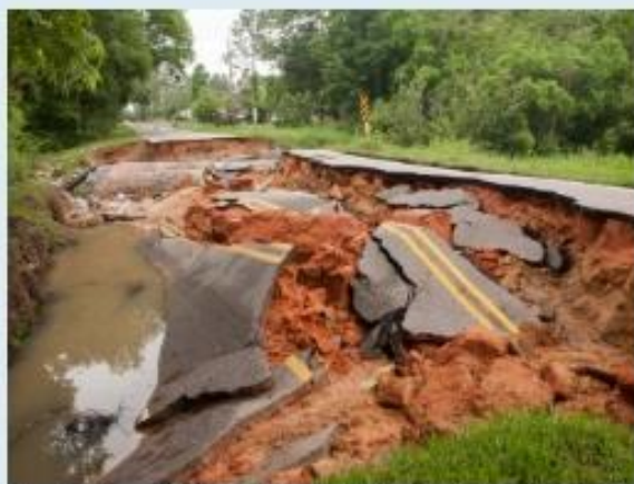
Flooding of a small stream in June 2014 destroyed this roadbed in Foley. Credit: Patsy Lynch, FEMA.
