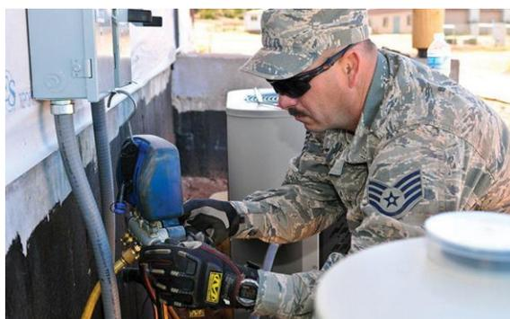
The emission of ODCs and greenhouse gases used for cooling and refrigeration are estimated using a mass balance approach. When a unit is worked on, often gas is removed from the unit prior to repairs. This gas is either reinjected into the unit after the repair is complete, reclaimed or disposed of. After the repair is complete, gas is added back to the system until the system has a full charge. The amount of
